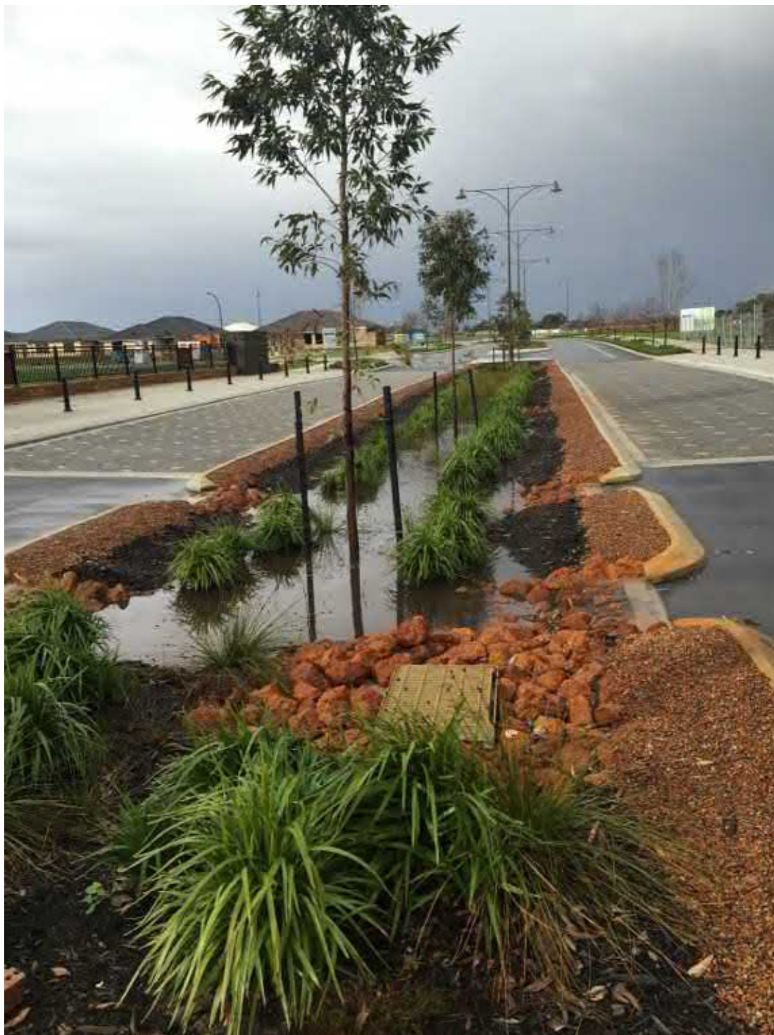
Figure 13: Typical median swale or biofilter
