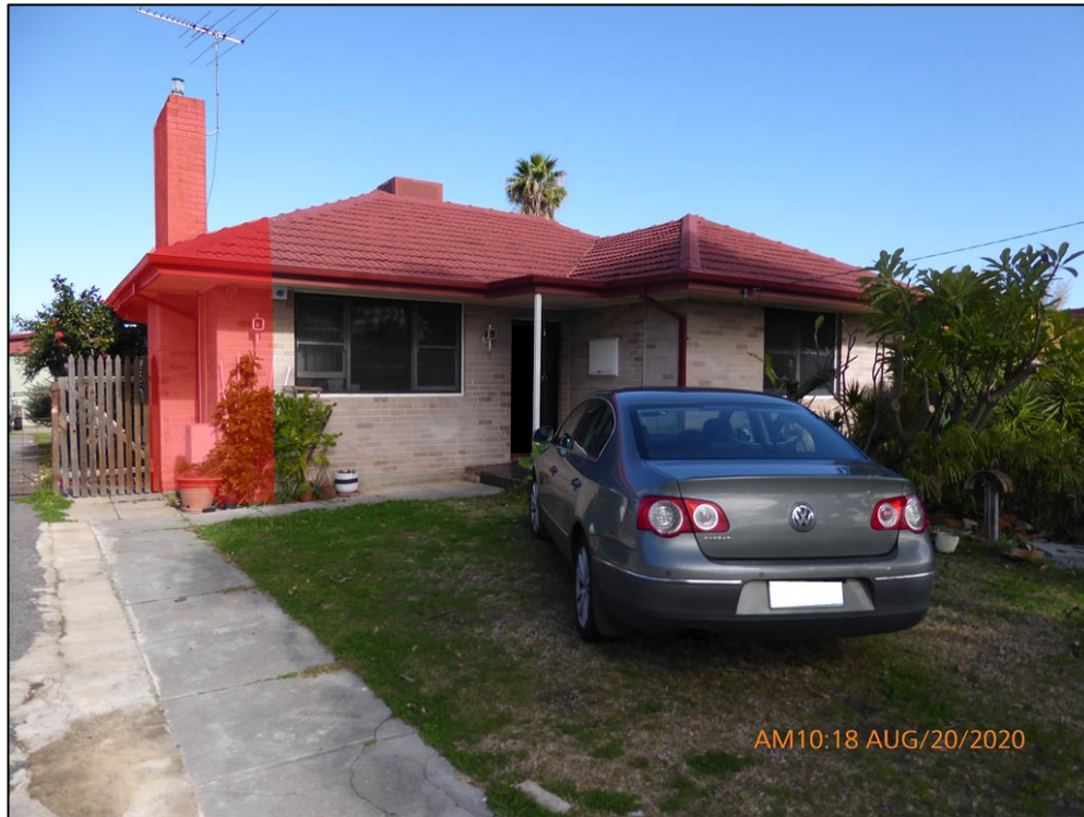
Figure 8: Portion of Existing House Requiring Demolition to Comply with Clause 5.7.3(c) of LPS 15
