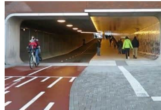
Figure 56: Safe, convenient and attractive underpass opportunities.
