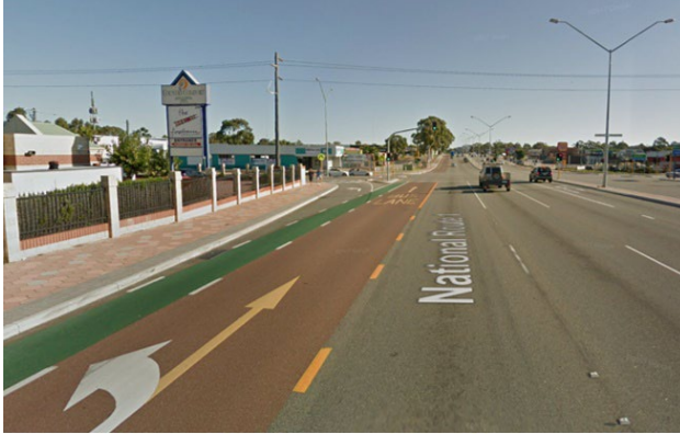
Figure 16 Typical bike lane arrangements along the Great Eastern Highway corridor (source: Nearmap and Google Streetview)
