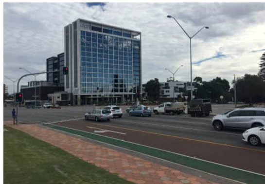
Figure 53: Safe and convenient at-grade pedestrian crossings
