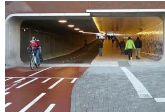
Figure 56: Safe, convenient and attractive underpass opportunities.
