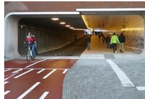
Figure 56: Safe, convenient and attractive underpass opportunities.
