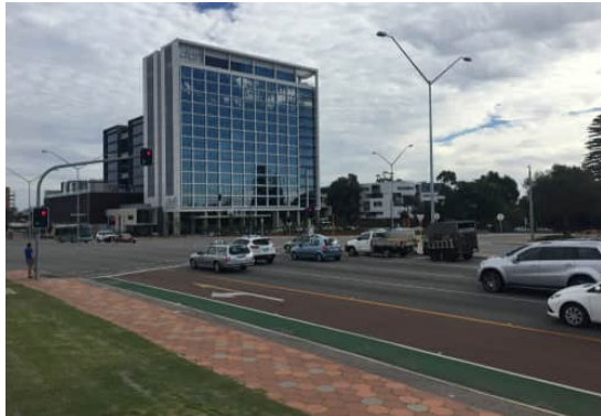
Figure 53: Safe and convenient at-grade pedestrian crossings
