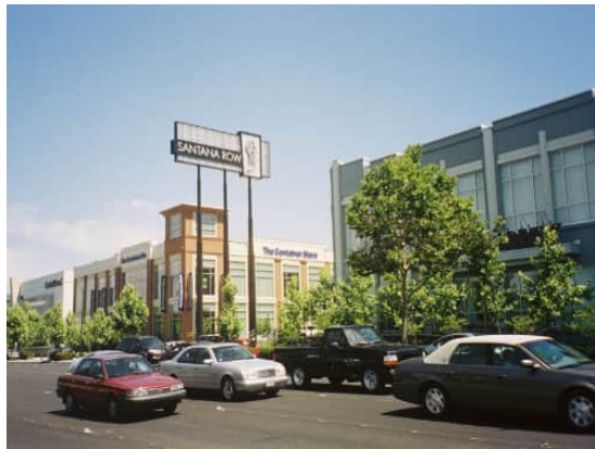
Figure 62: Well-articulated development relating to the street edges
