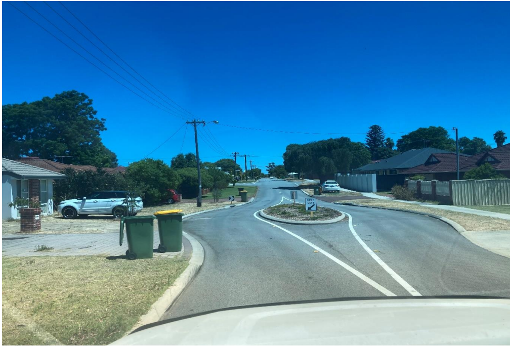
Lyall Street: Existing Slow Point west of Victoria Street.
