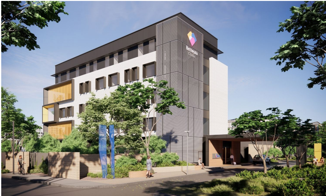
Figure 5. Cockburn Mental Health Hospital, Cockburn Central West
