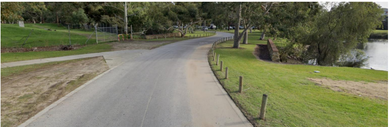
Figure 21 – Cross section of Memorial Dr west of Stoneham St, looking east (source: Google Street View)
