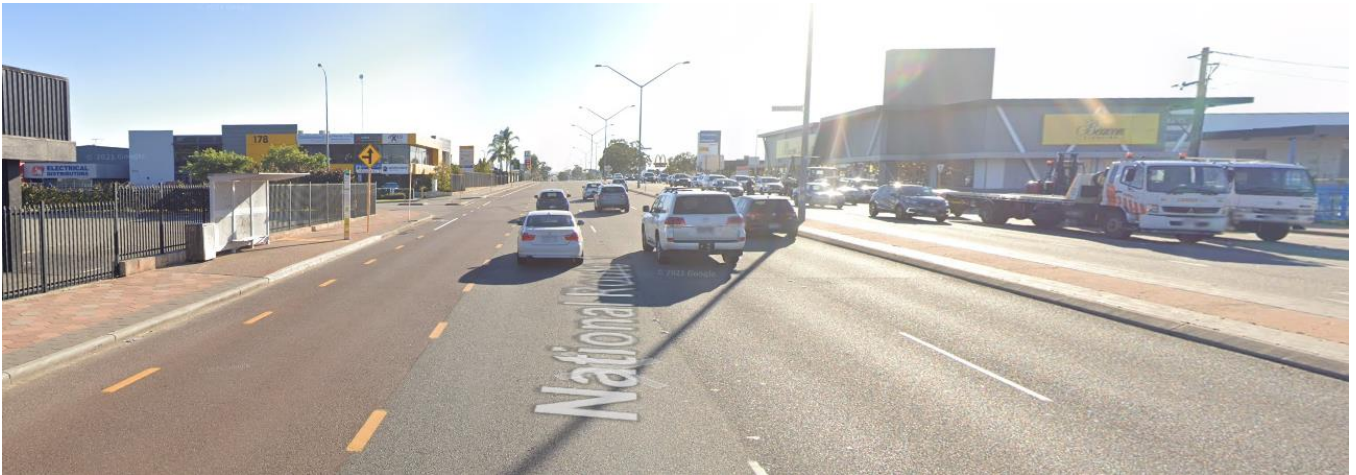
Figure 12 – Cross section of Great Eastern Highway corridor– looking east, west of Hargreaves St (source: Google Street View)
