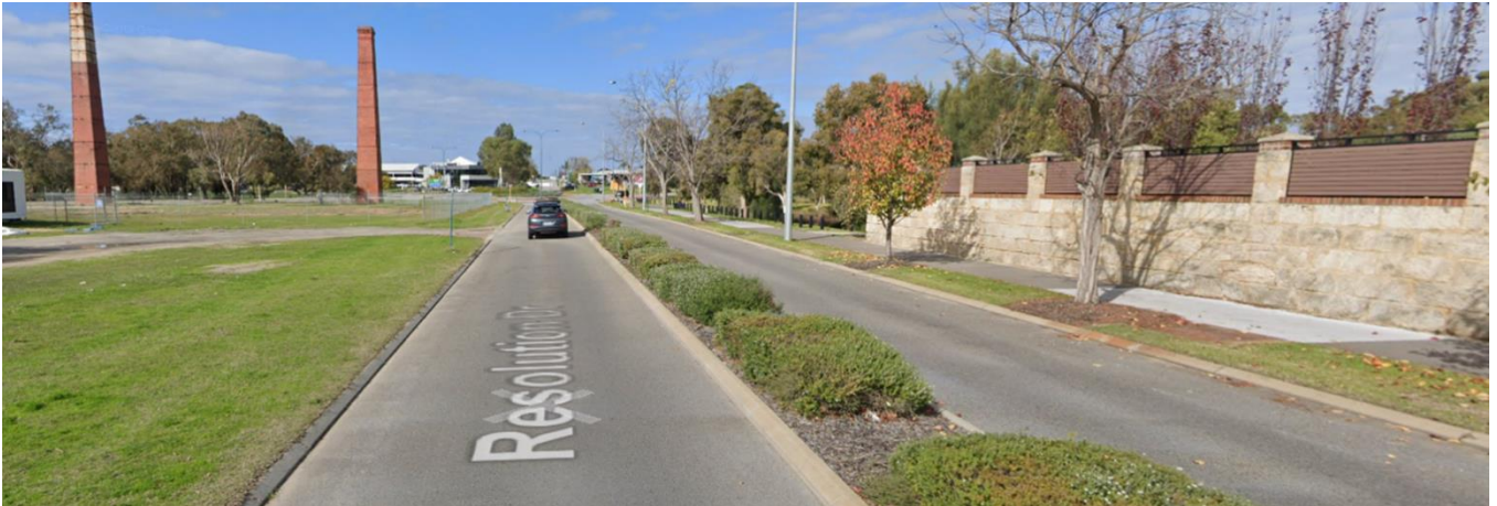
Figure 20 – Cross section of Resolution Dr (northwest) north of Stoneham St, looking south (source: Google Street View)
