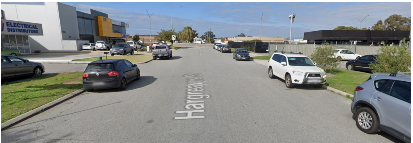
Figure 17 – Cross section of Hargreaves St, north of Great Eastern Hwy, looking south (source: Google Street View)
