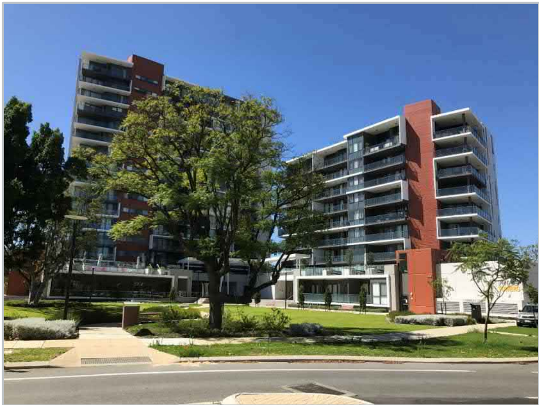
Figure 5 - Example of Development on Great Eastern Highway
