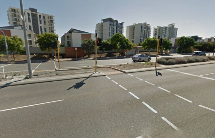
At-grade two-stage pedestrian crossing facility. With pedestrian call buttons in the central median
