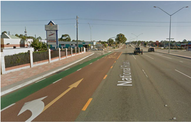
Figure 16 Typical bike lane arrangements along the Great Eastern Highway corridor (source: Nearmap and Google Streetview)
