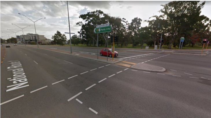
At-grade pedestrian crossing – requiring pedestrians to cross 8 lanes (38m) in a single movement. No pedestrian call button in the central median
