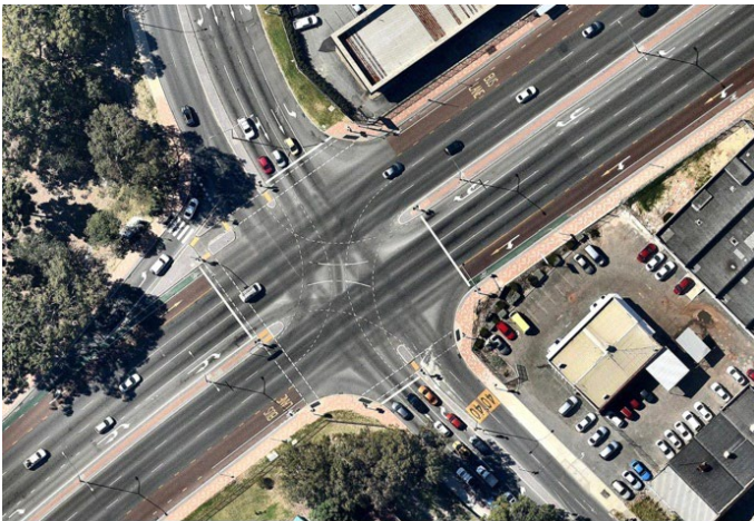
Figure 19 Typical bus lane arrangements at traffic signal intersections along the Great Eastern Highway corridor (source: Nearmap)
